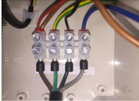
Do not force large diameter TPS cable's wires into the block without sleeves, or the block may overheat due to a poor connection.
